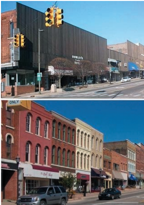
Figure 53: Renovation Completed by MN Main Streets Program
