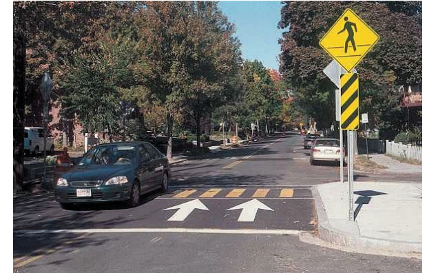
Figure 42: Traffic Calming Using Speed Hump at a Crosswalk
