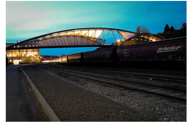
Figure 36: Example of Pedestrian Bridge Over Railroad Tracks
