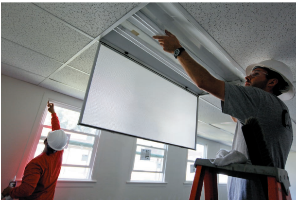
Figure 59: Installing New Energy Efficient Lights
