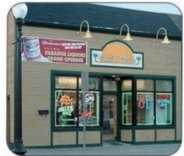
Figure 52: Facade Renovation- Before and After
